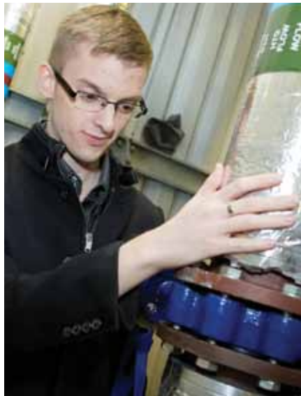
Gray checks for hot valves in the CHP plantroom
